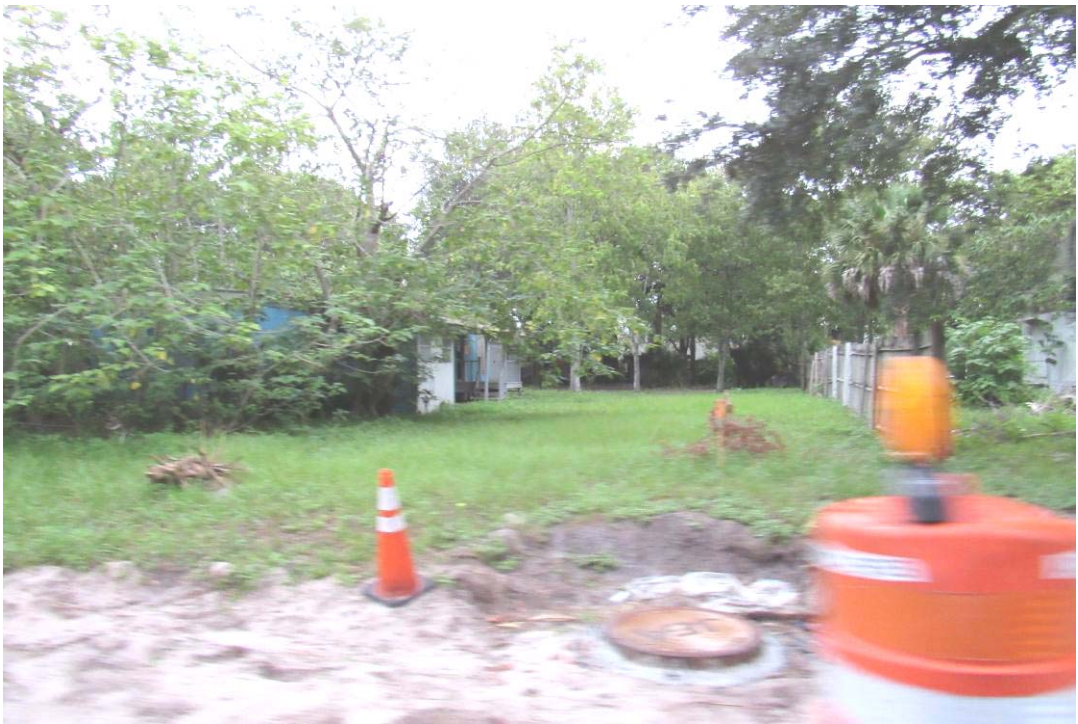
View of subject site.
